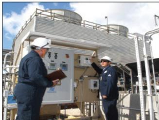
Figure 5. This image shows the 3D Trasar technology set up on a cooling tower.
