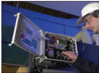
Figure 4. A technician looks inside a 3D Trasar Controller, which helps maintain control over critical cooling assets
